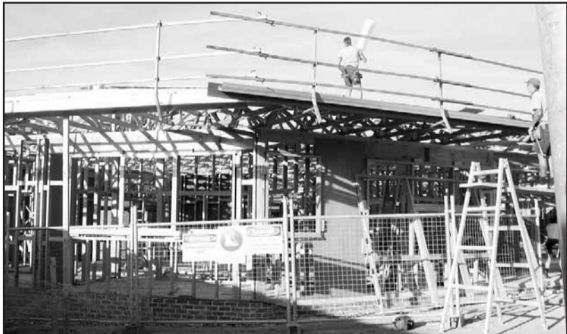
Progress of our new Library and Technology centre
