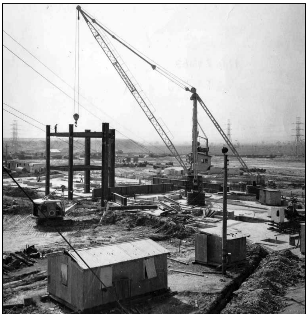
The first steel frame erected for the power station building
