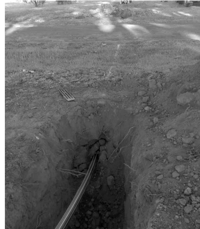
The new water pipe at the Hazelwood Cemetery.
