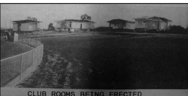
CLUB ROOMS BEING ERECTED
