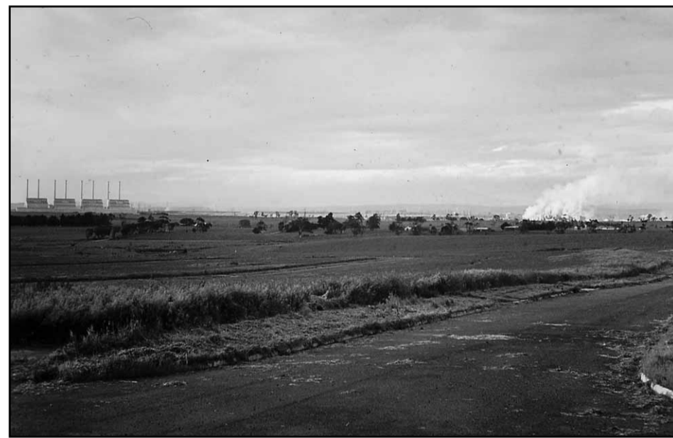
Early construction looking towards Hazelwood Power Station
