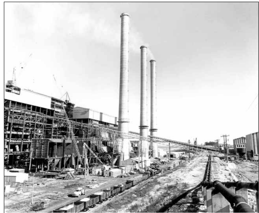
The construction of Hazelwood Power Station
