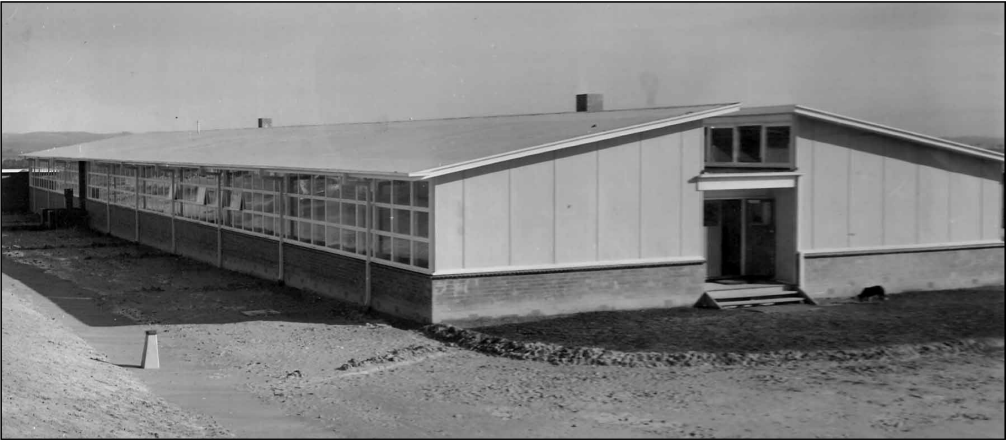
Construction of Churchill Primary School
