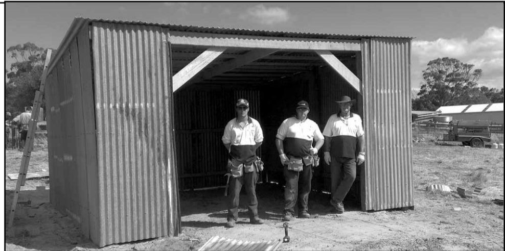
The horse shed built by the VCAL students
