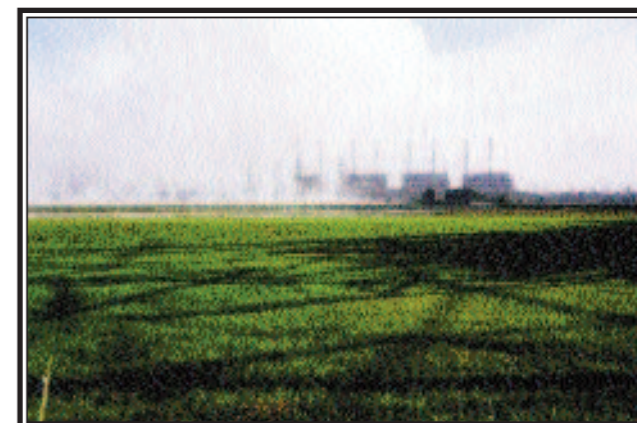
HAZELWOOD POWER STATION
