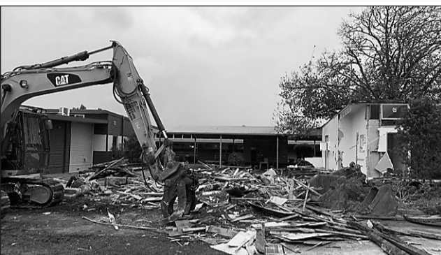
Demolition of the old administration block
