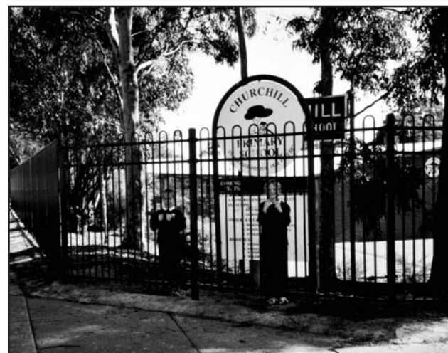
The new fence
