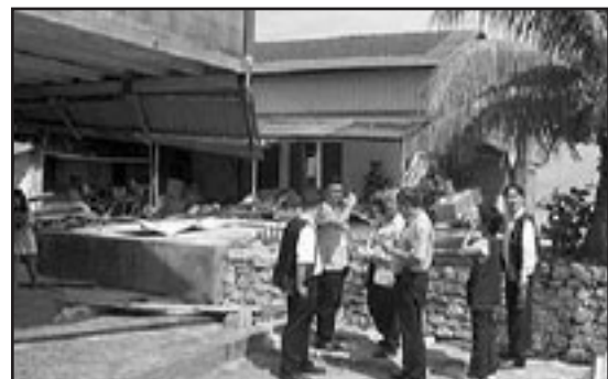
LCIF Tsunami Rebuilding Project – inspecting the damage
