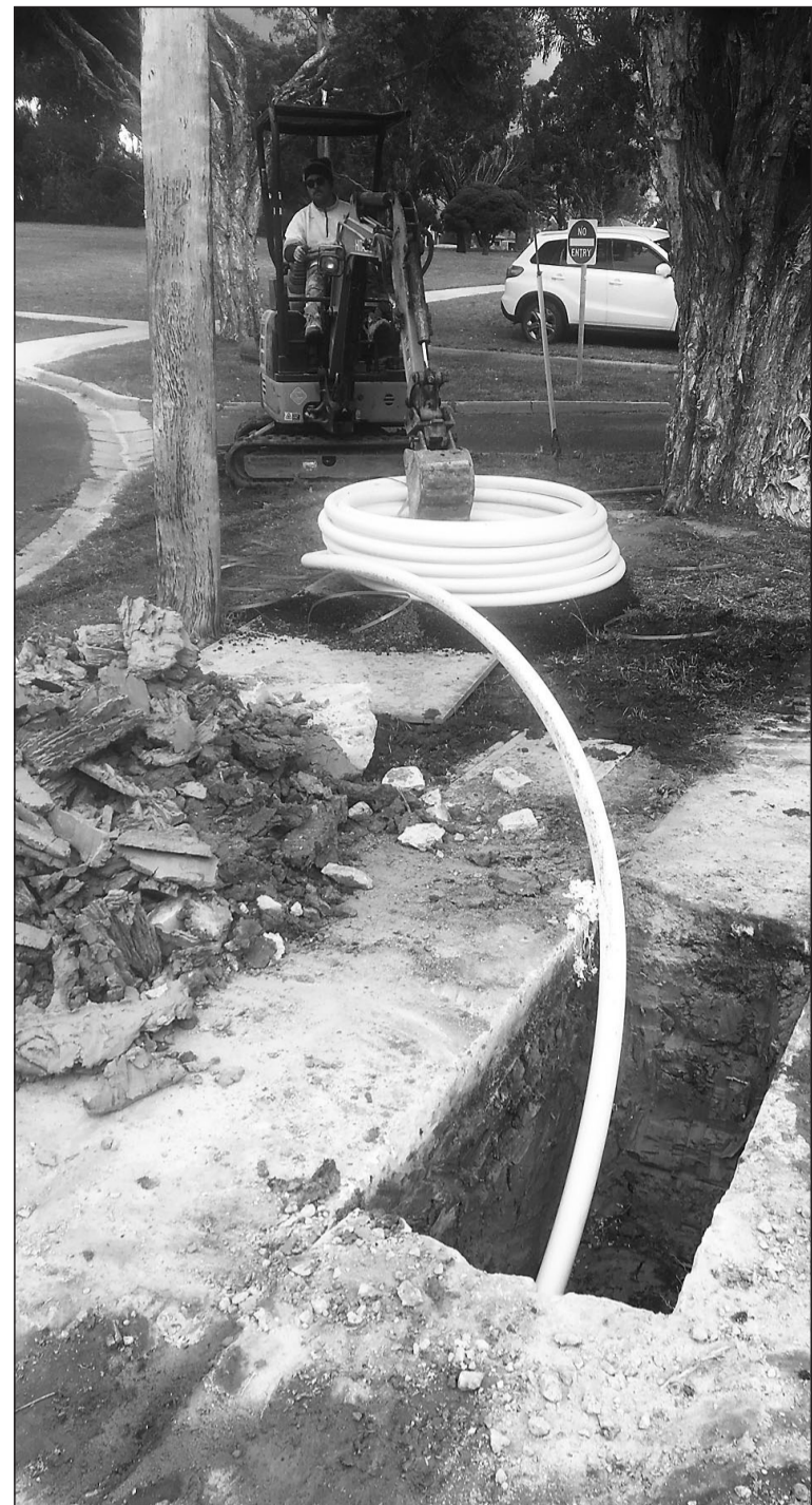
Left - Drilling machine at work
