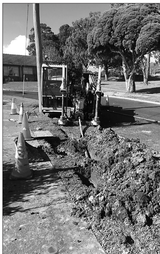
Above - the pipe being threaded through the drilled hole as the drilling machine withdrew from the space
