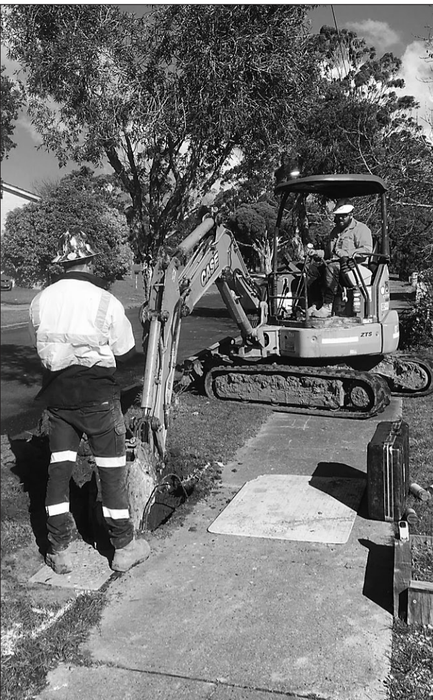
Excavator digging holes
