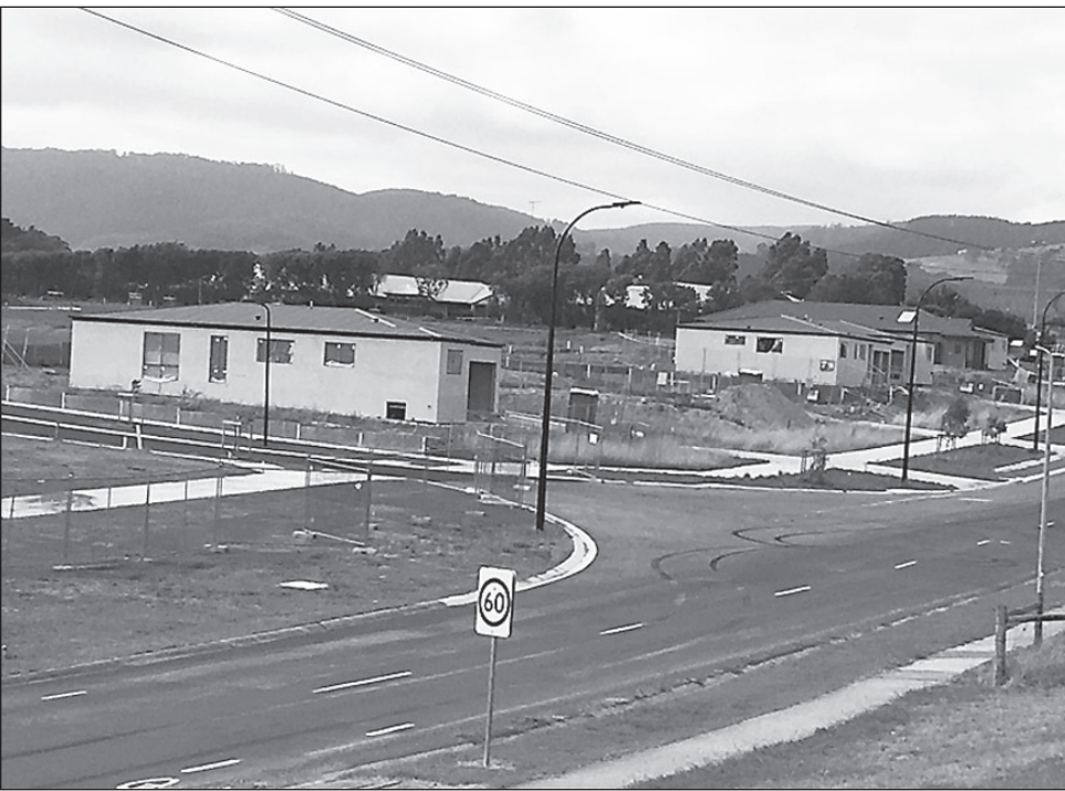
More houses being built in and around Churchill
