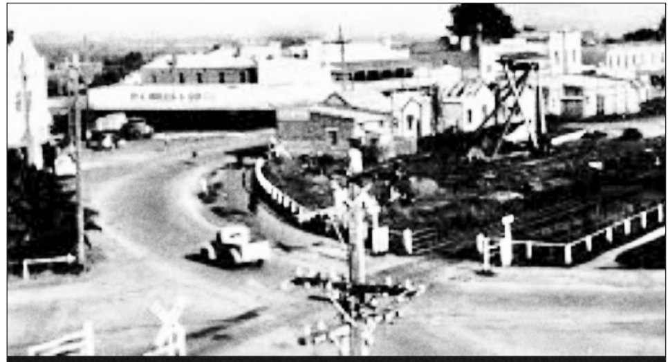
The accompanying photograph circa early 1930's shows the infamous at-grade Morwell railway crossing. Railway crossing signage had improved by then, but note the rail tracks at street level
