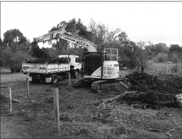
Willows being removed
