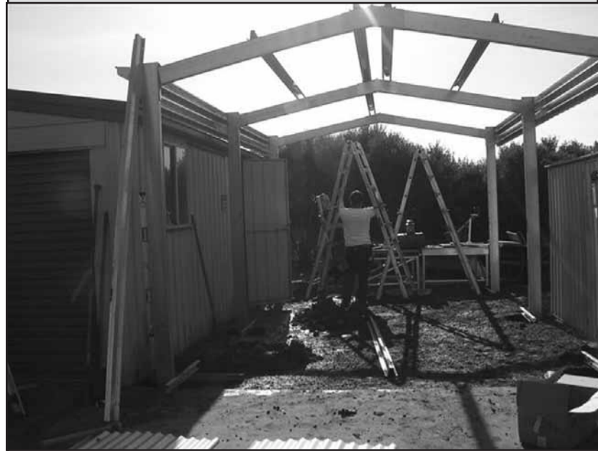
The new carport for the hostel bus almost nearing completion
