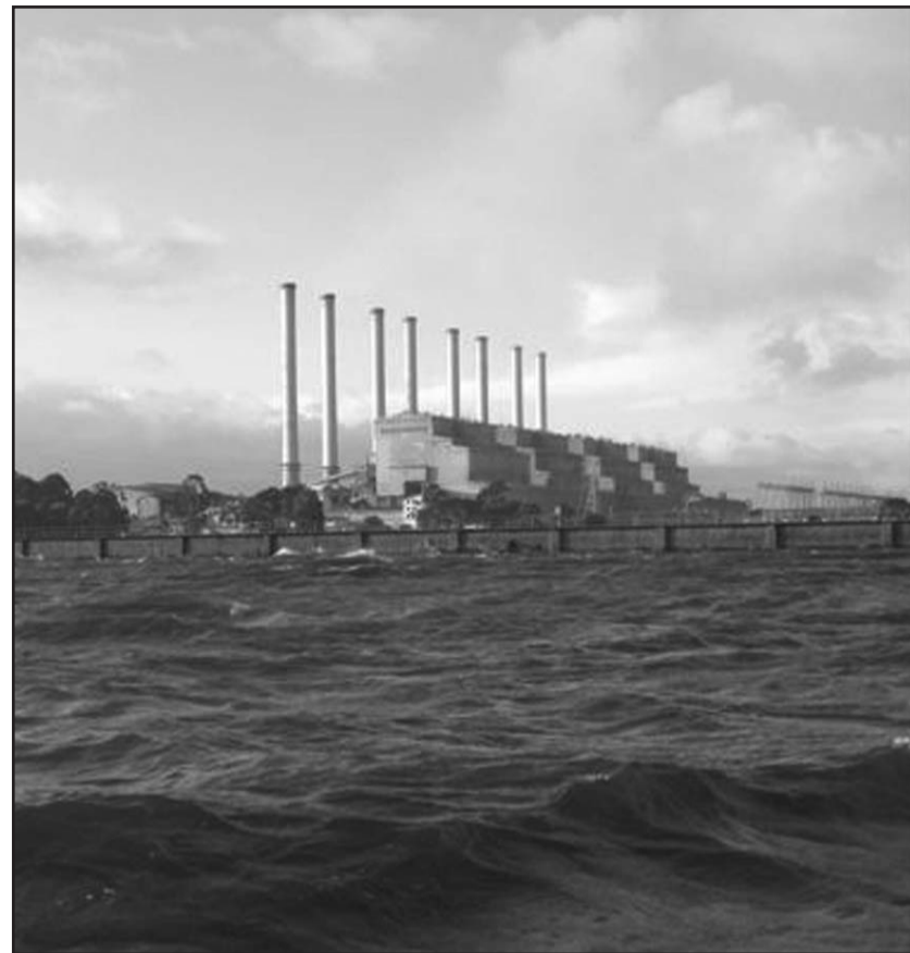
Hazelwood Power Station
