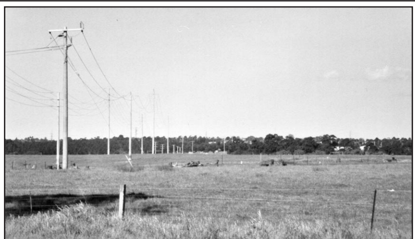
Site of the new Strzelecki Highway - from Marretts Road looking north east to Morwell
