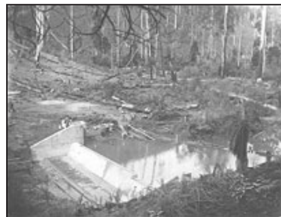
Pictured top left: Early photo of the Weir - c.1914, above top: Billys Creek Weir c.1949, above: Weir under construction c.1913
