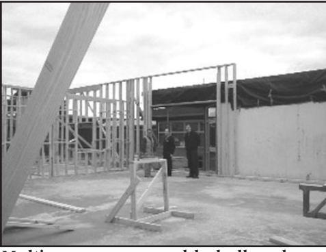
Multi-purpose assembly hall under construction
